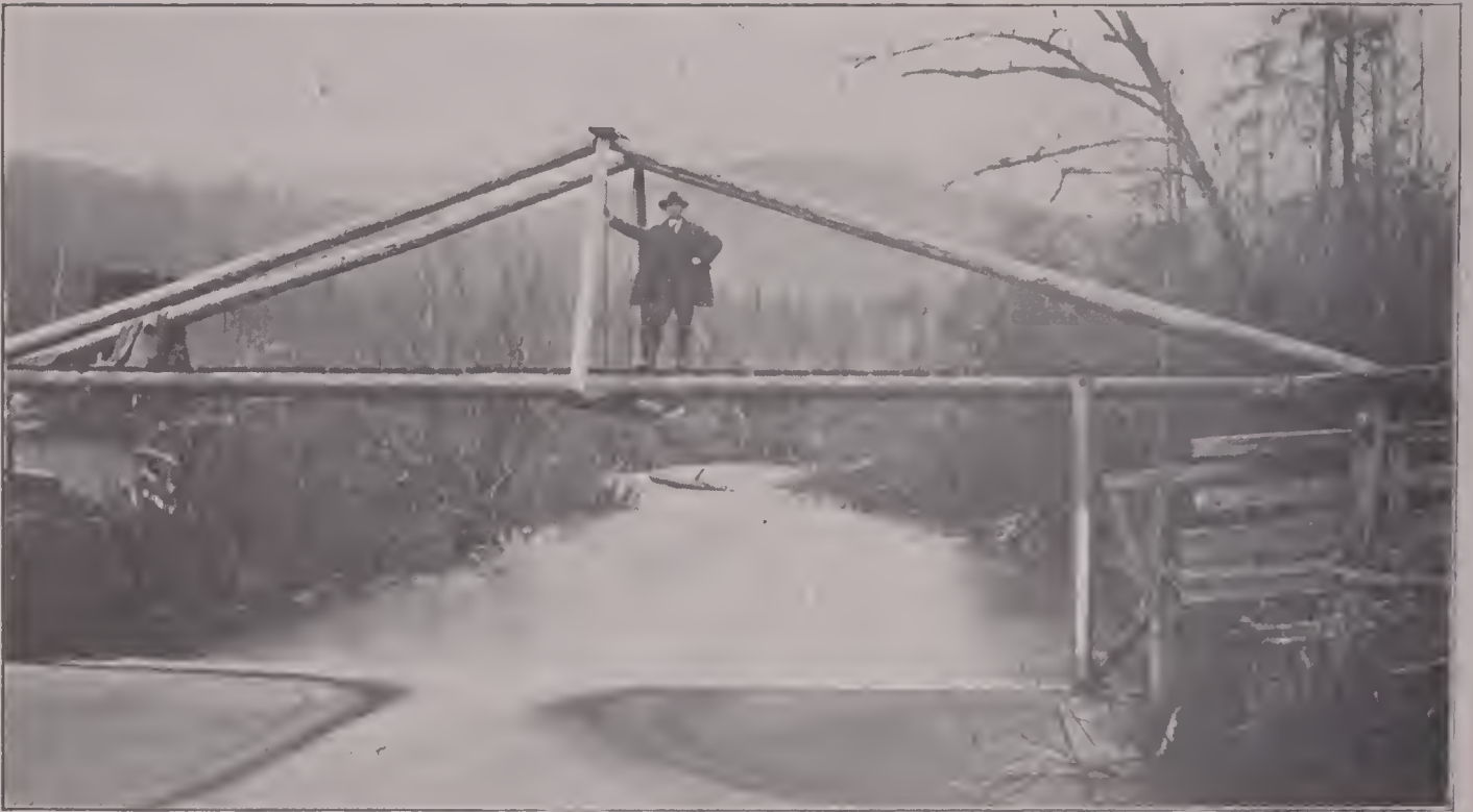
A ARTIFICIAL CONTROL AND GAGING BRIDGE, EAST CREEK NEAR ELBE.
